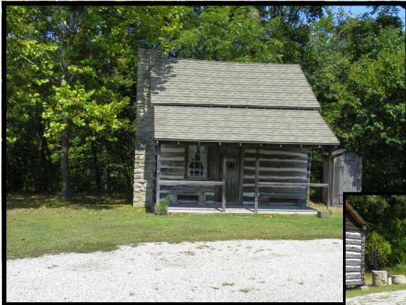
A new metal roof was put on the Lupardus cabin.
